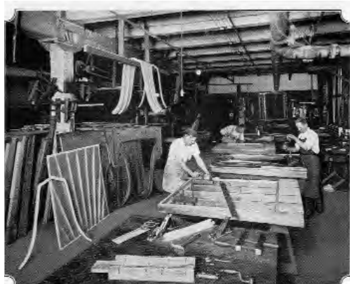
The manufacturing process at the Mills factory in Chicago: Making the piano backs and sounding boards. (This and the following pictures are from Building the Violano-Virtuoso )
